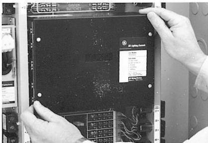
Insert the RCC48 Controller Card and associated RRDC12 Relay Driver Cards.
