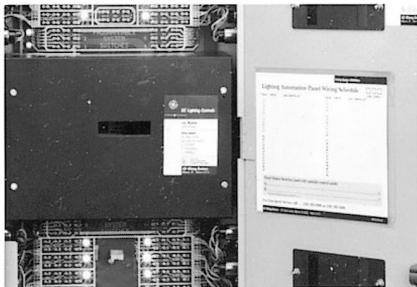
Check the RCC48 Hardware Status LED (to the right of the Panel Address setting knobs): Off = No power; On steady = Okay; Flashing = Defective board.
