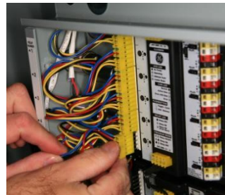
Relay #1 - #6 connection to first relay module
