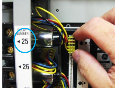
Relay #25 - #30 connection to fifth relay module
