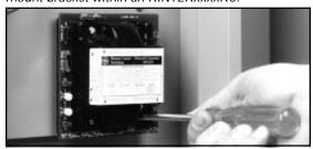
Connect Low-Voltage Wiring. Wire to the 24 VAC power supply and connect Red (ON) and Black (OFF) outputs to the corresponding inputs on the relays to be controlled.
