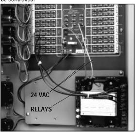
**Connect Photosensor.** Connect the Red/Black/Blue/ White wires from the sensor to the corresponding RPCON photocell terminations.
