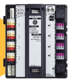
The **CLCDIM4 dimming module** controls four dimming channels. Through the color-coded spring terminals, the device provides 0-10V dimming controlled by a photocell for daylighting operations, as well as advanced scene control via devices in the CLC network.
