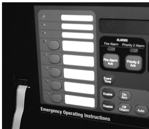
Figure 3-10. Connecting Serial Cable
